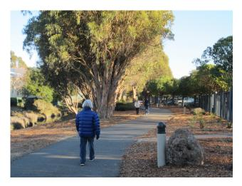
Restore the DG shoulder to within two feet of the lighting bollards on the inland of this Meeker Tidal Creek Trail. On the creek side, restore and widen the shoulder to six feet where feasible without incurring excessive cost. The shoulder will narrow to less than six feet in places due to lack of usable space between the AC pavement and the creek or the presence of massive eucalyptus trees.
